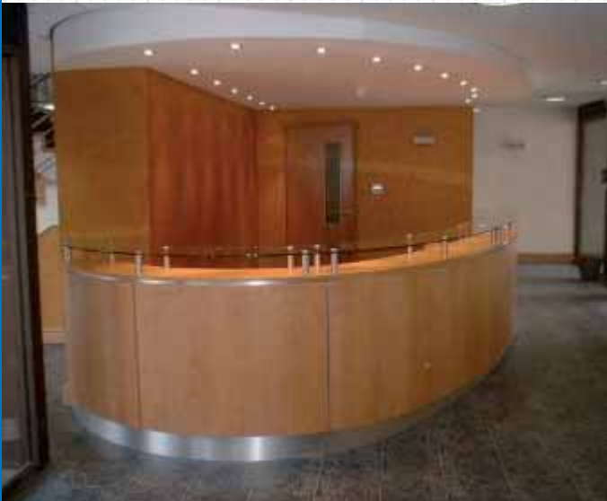
Curved reception counter wood grain carcass and a laminated worktop.
